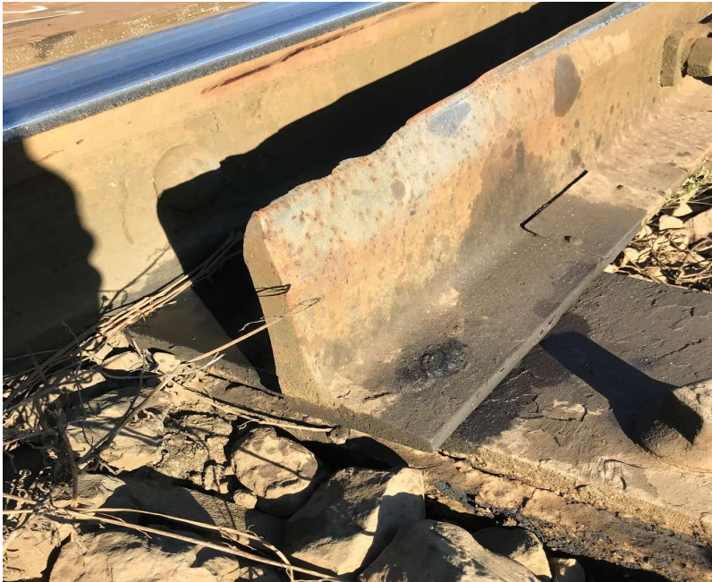
Before Assessed Condition Code 4
