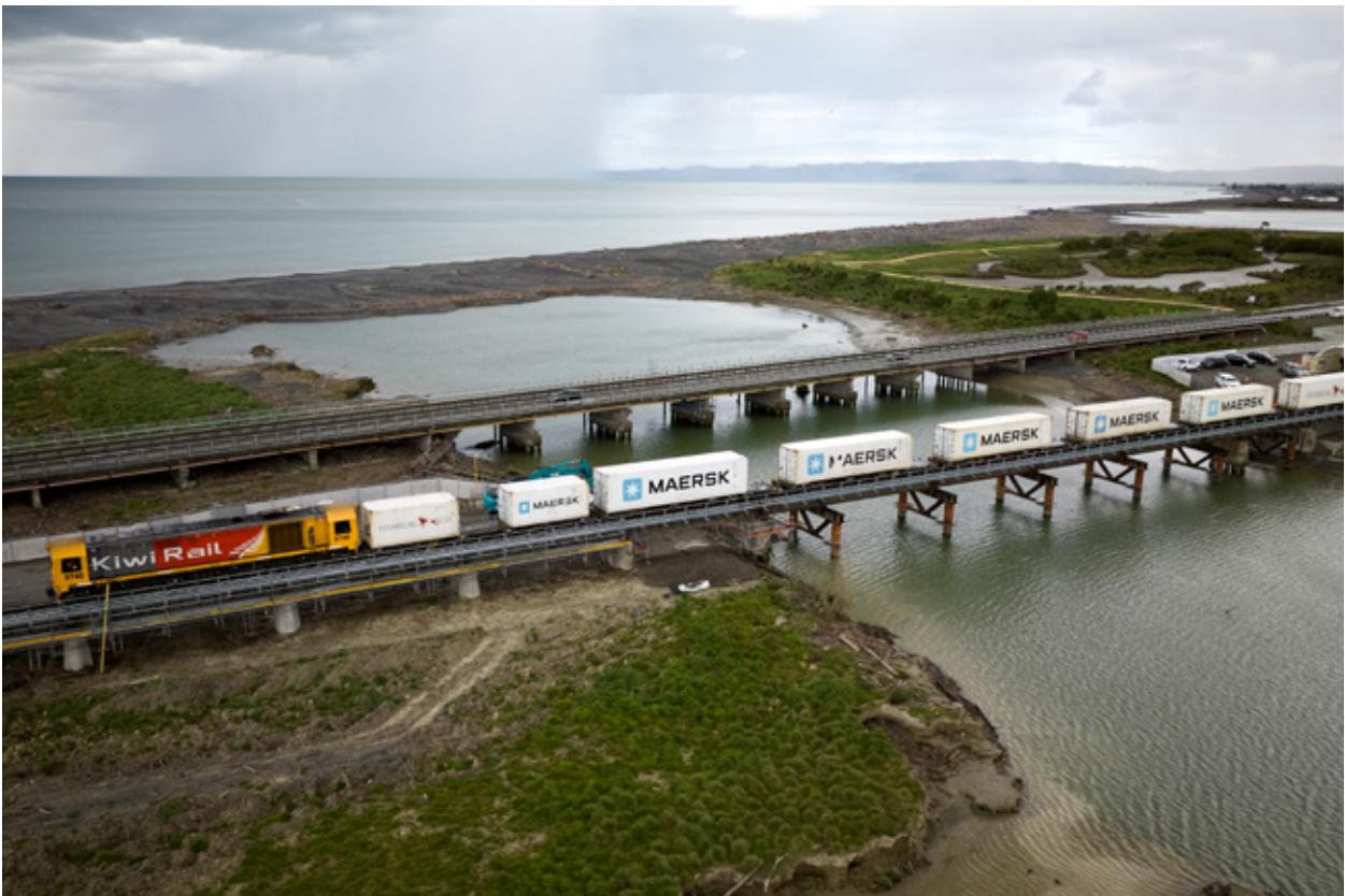
Cyclone Gabrielle closed the line between Hastings and Napier in February with track and embankments washed away, and major damage to Bridge 217, which lost piers and spans in the floods. KiwiRail teams worked hard to restore the line, replacing 800 sleepers, 140 metres of rail, laying 3,000 cubic metres of formation (the rock foundation under the tracks) and 3,500 tonnes of ballast.
